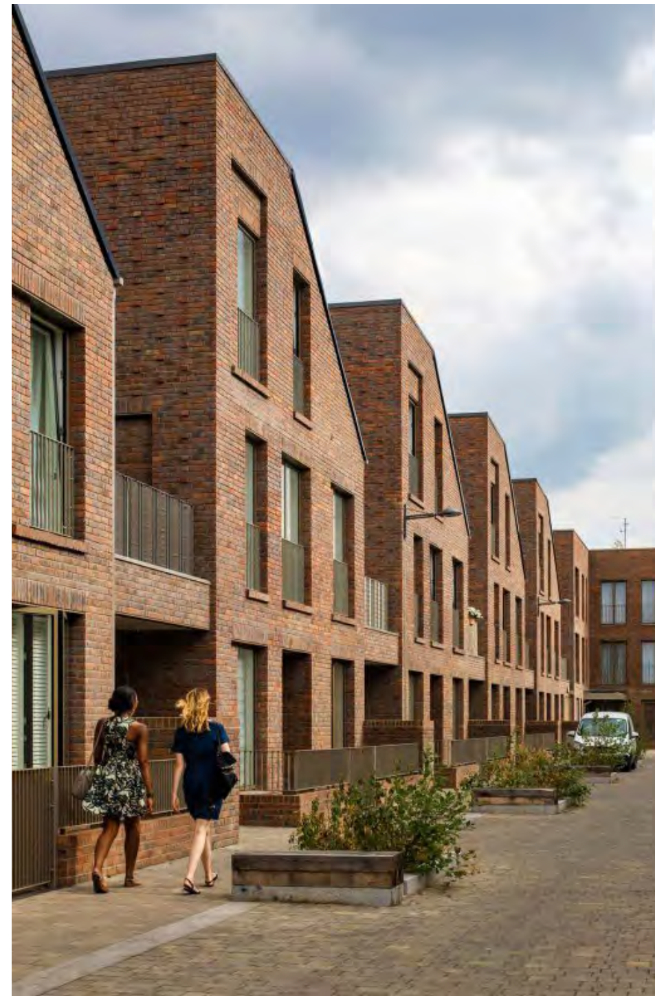
High quality family homes and streetscape – Dujardin Mews, Enfield
