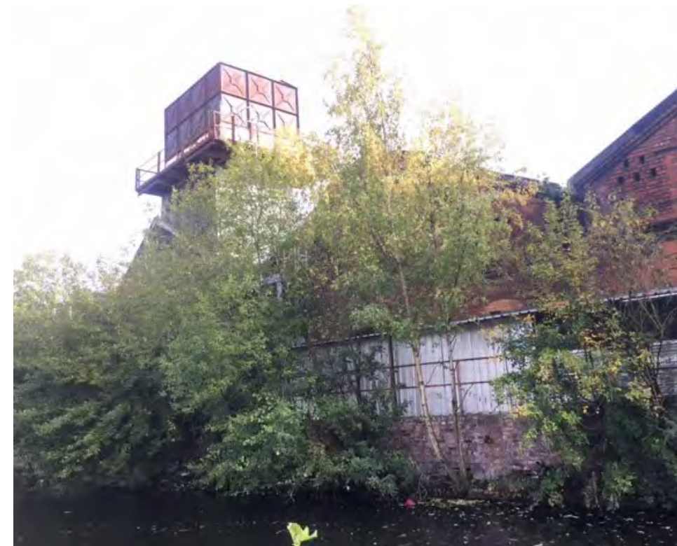
Existing water tower
