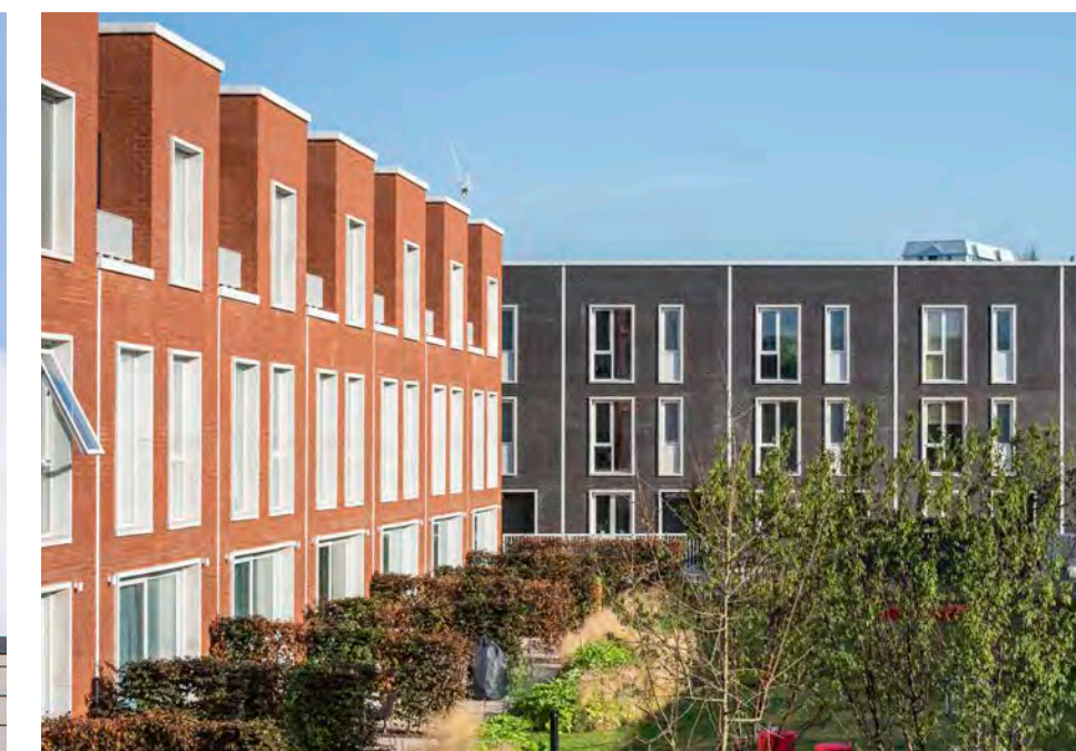
Materiality at Port Loop, Birmingham
