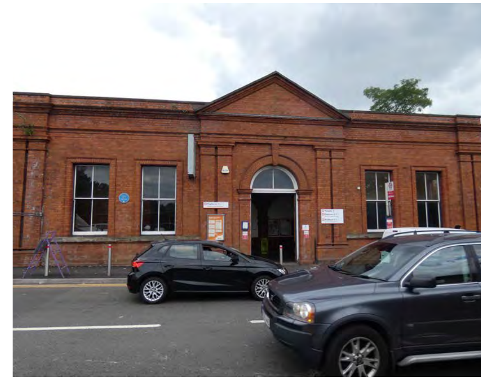
Rolfe Street station building
