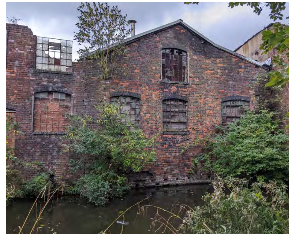
Existing warehouse elevations onto the Engine Arm
