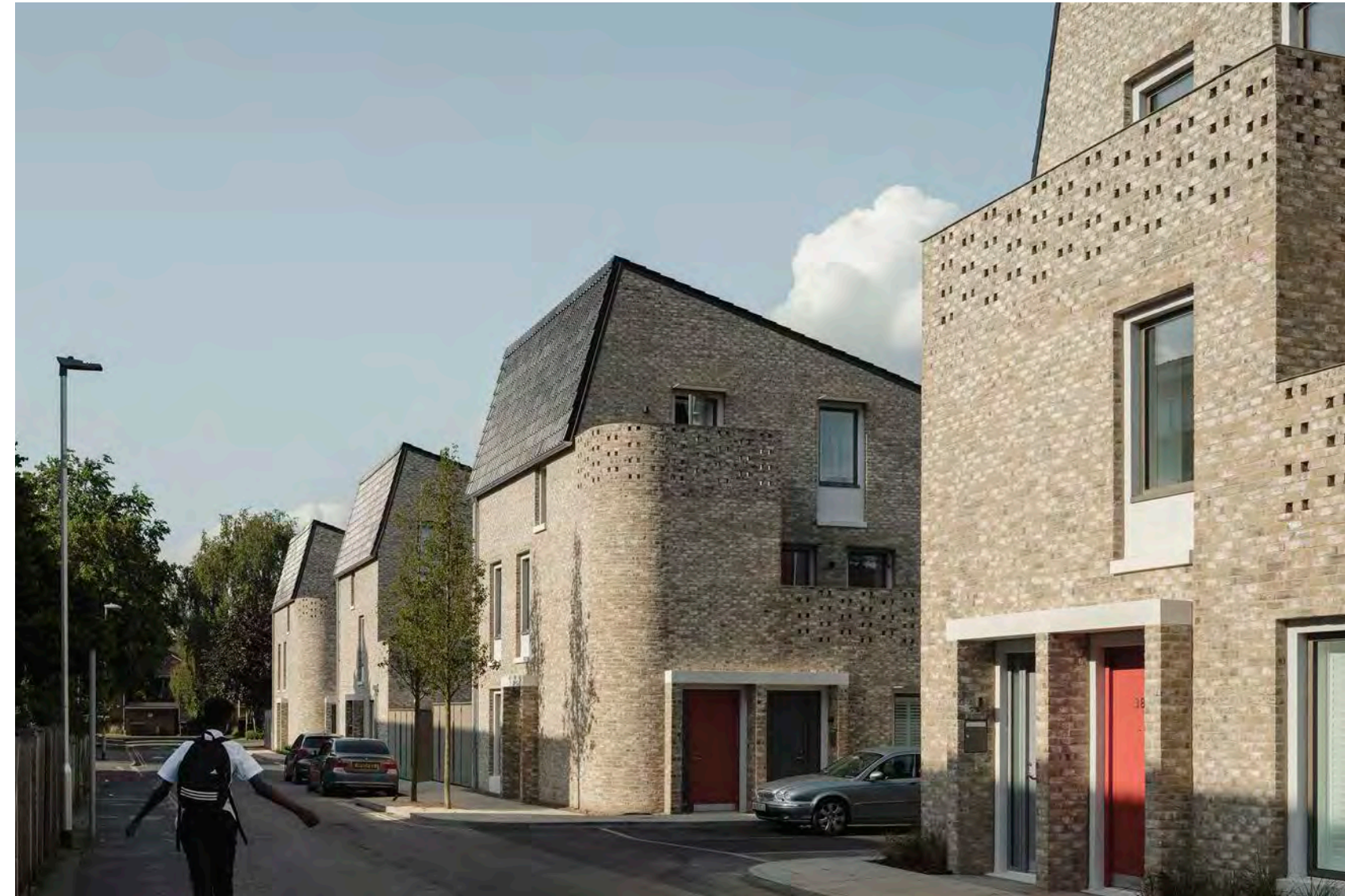
Triplex corner apartments with own front door: Goldsmith Street, Norwich
